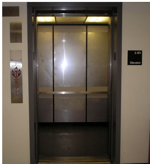
Figure 4. Taylor building elevator
