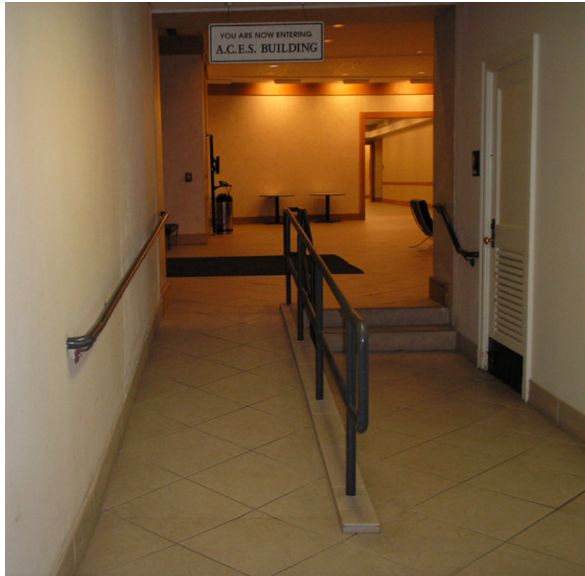
Figure 5. Taylor/ACES wheelchair ramp
