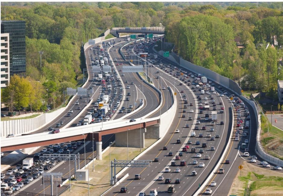
*The relatively new Express (HOT) Lanes in the center of I-495 in Northern Virginia with an exclusive grade-separated on- and off-ramp. (Photo: Courtesy of TransUrban)*
